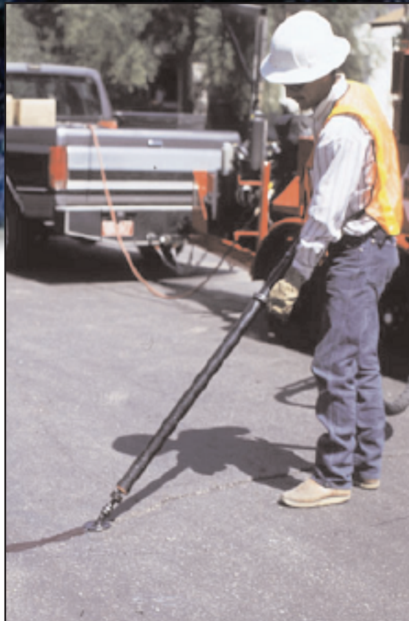
Placing crack sealant.
