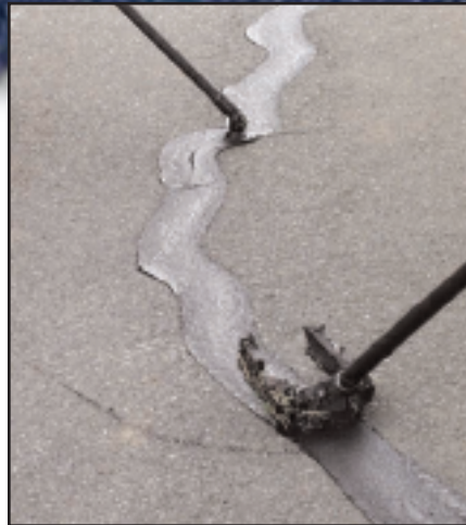
Using squeegee to install sealant.
