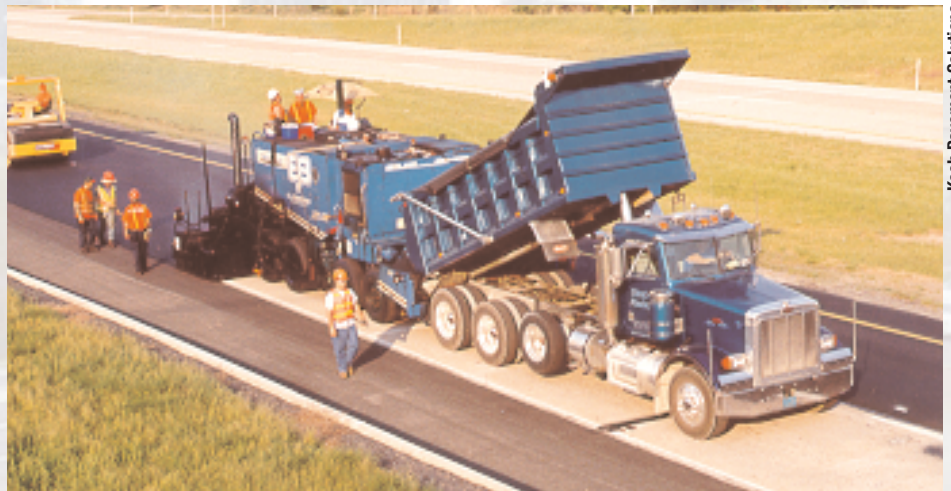
Constructing a thin, bonded overlay.
