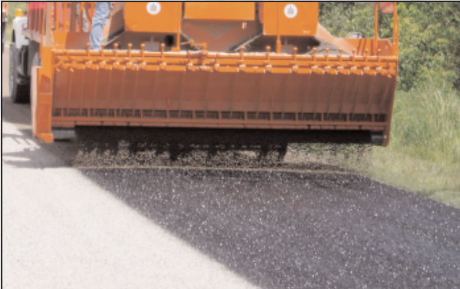
Constructing a chip seal.
