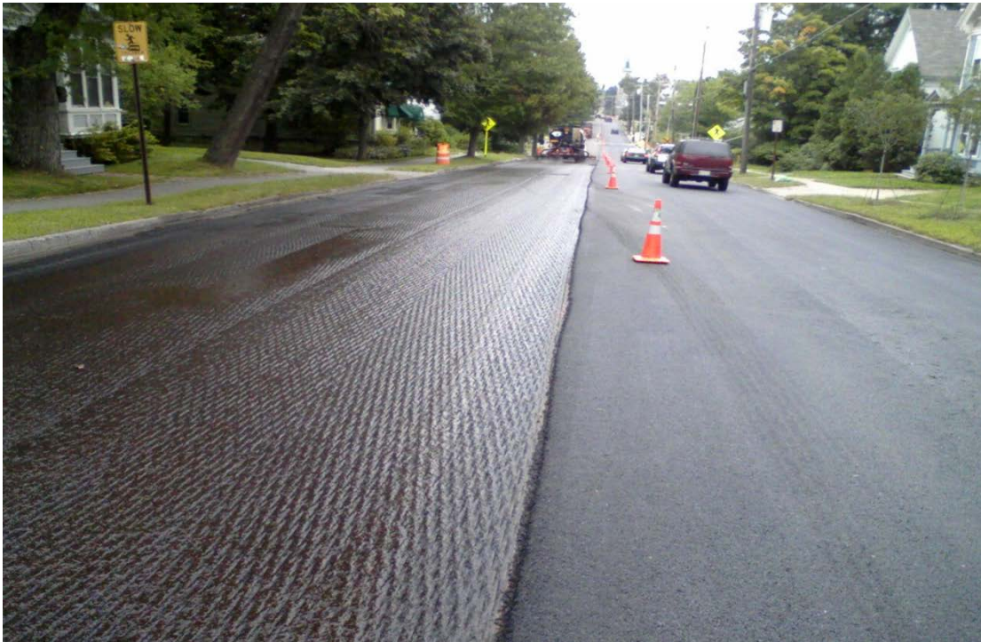
Figure 5. A uniform tack application.
