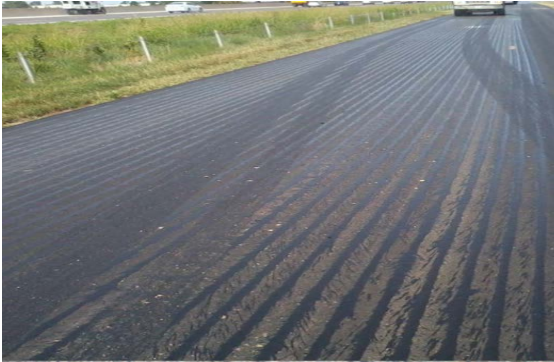
Figure 5. A uniform tack application.
