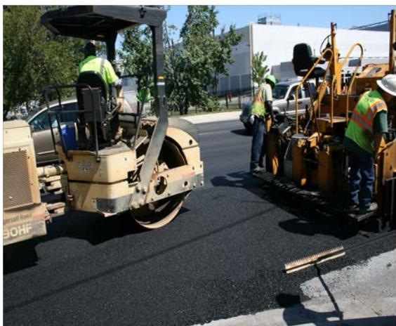
*Keeping the rollers close to the paver is always important, it is critical when the weather turns cool/cold.*
