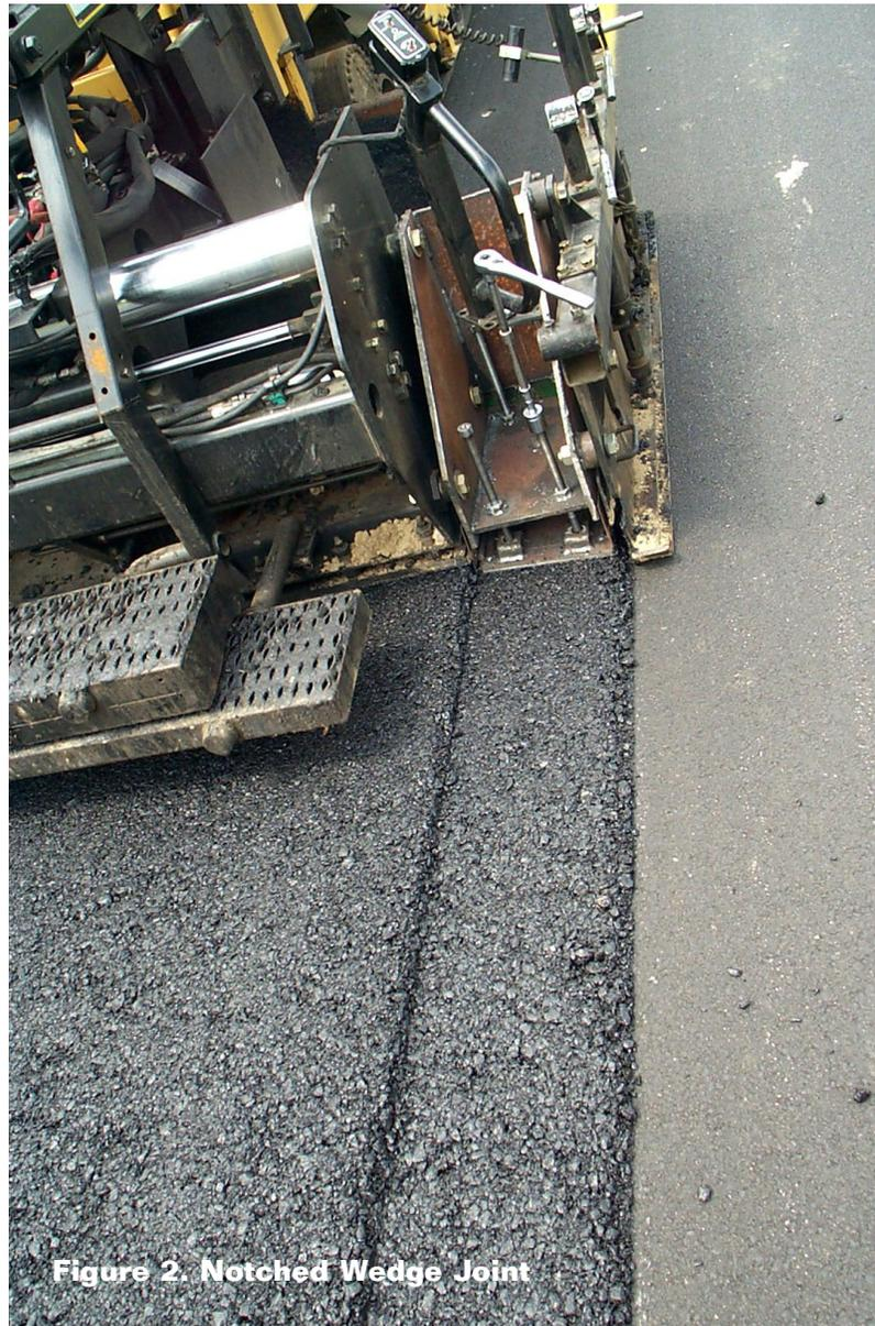
**Figure 2. Notched Wedge Joint**
