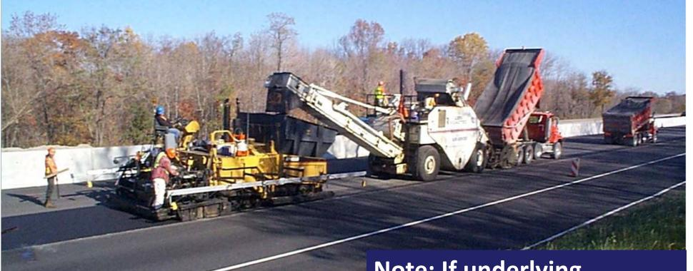
Versus Joint Matcher, which is best for joint (reference is exact location just in front of auger) Note: If underlying pavement already smooth, some contractors feel they can get good joint with ski, but must finish 1/10" high
