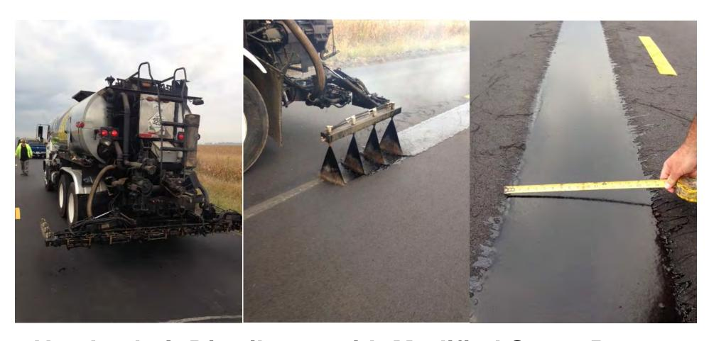
Hot Asphalt Distributor with Modified Spray Bar
