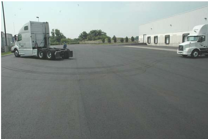
Same pavement showing truck traffic to loading docks the morning after paving.
