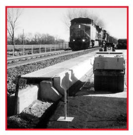
(HTL) of the Facility for Accelerated Testing (FAST) track. A pit approximately 700 feet long, 12 feet wide and 5 feet deep was excavated in the subgrade beneath a section of existing track. The intent of the experiment was to model the effect of a low modulus subgrade on track modulus and geometry.
