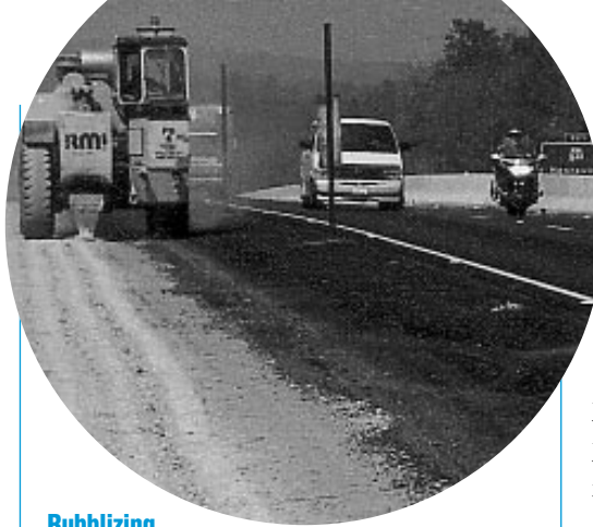
Rubblizing close to traffic on I-65 in Alabama.
