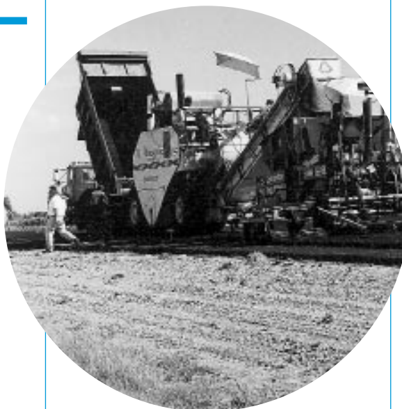
Overlaying the rubblized mainline on I-65 in Indiana with 13.5 inches of Superpave mix.
