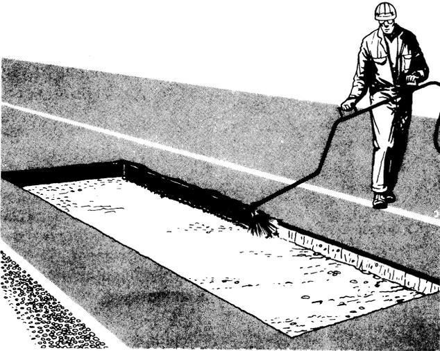
Figure II—Applying tack coat to vertical surfaces
