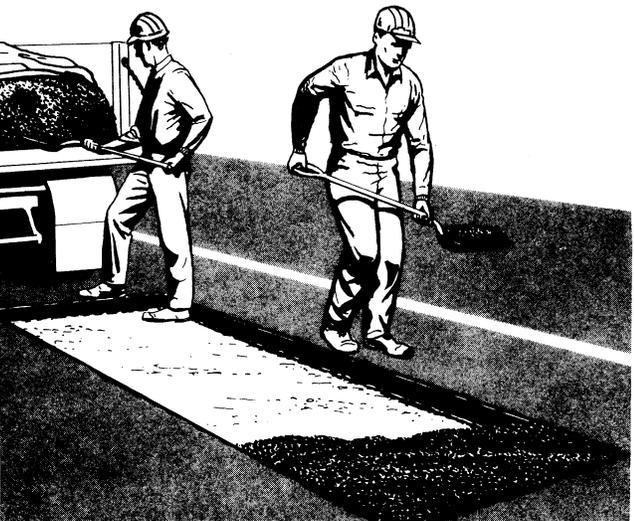
Figure III—Backfilling hole with plant-mix
