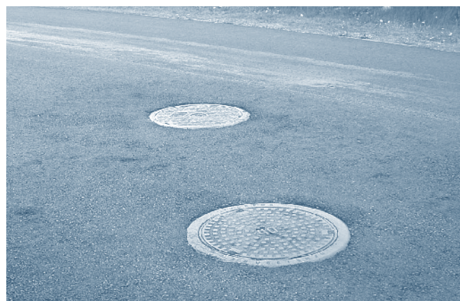
Figure 19. Handwork with WMA around manhole.
