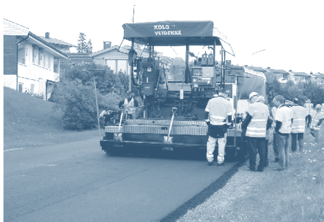
Figure 17. Heavy tamping-bar paver.
