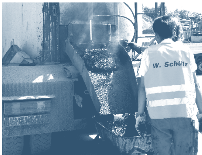
Figure 20. Unloading a mastic asphalt transport.
