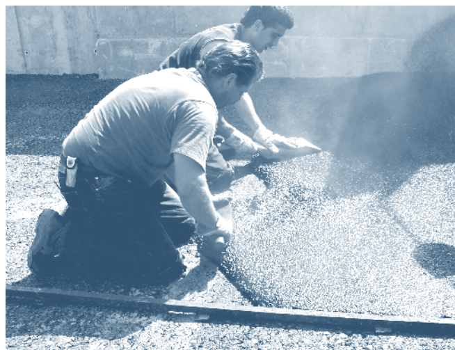
Figure 21. Placing mastic asphalt.
