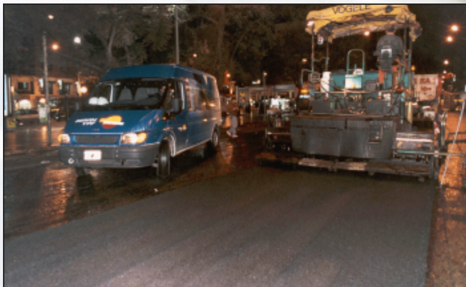
Placing the rubber modified asphalt.
