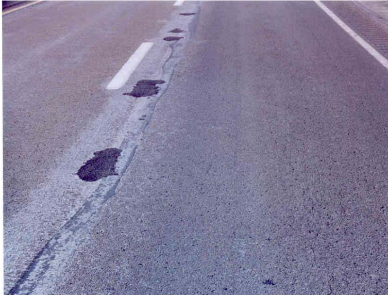
Figure 1. Deteriorating Longitudinal Joint
