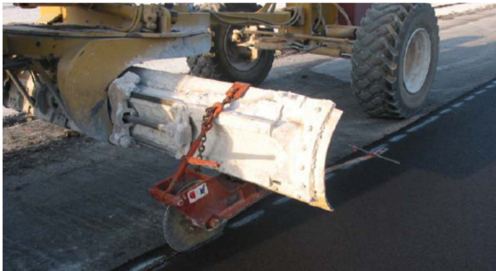
Figure 9. Cutting Wheel Attached to Grader for Airfield Project in U.S. (Prowell photo)
