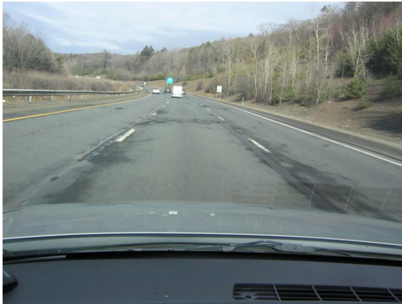
Figure 1. Deteriorating Longitudinal Joint
