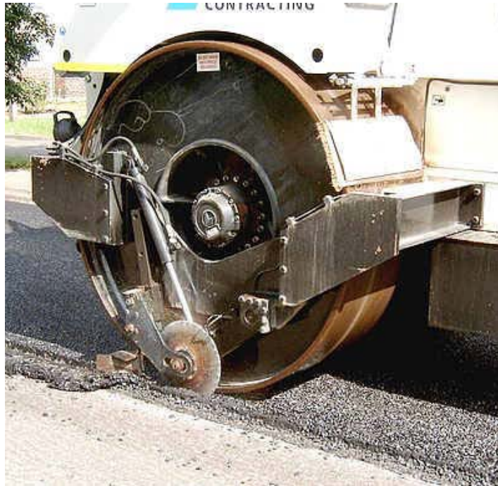
Figure 8. Cutting Wheel Fixed to Roller in the United Kingdom ( www.highwaysmaintenance.com/kraktext.htm )
