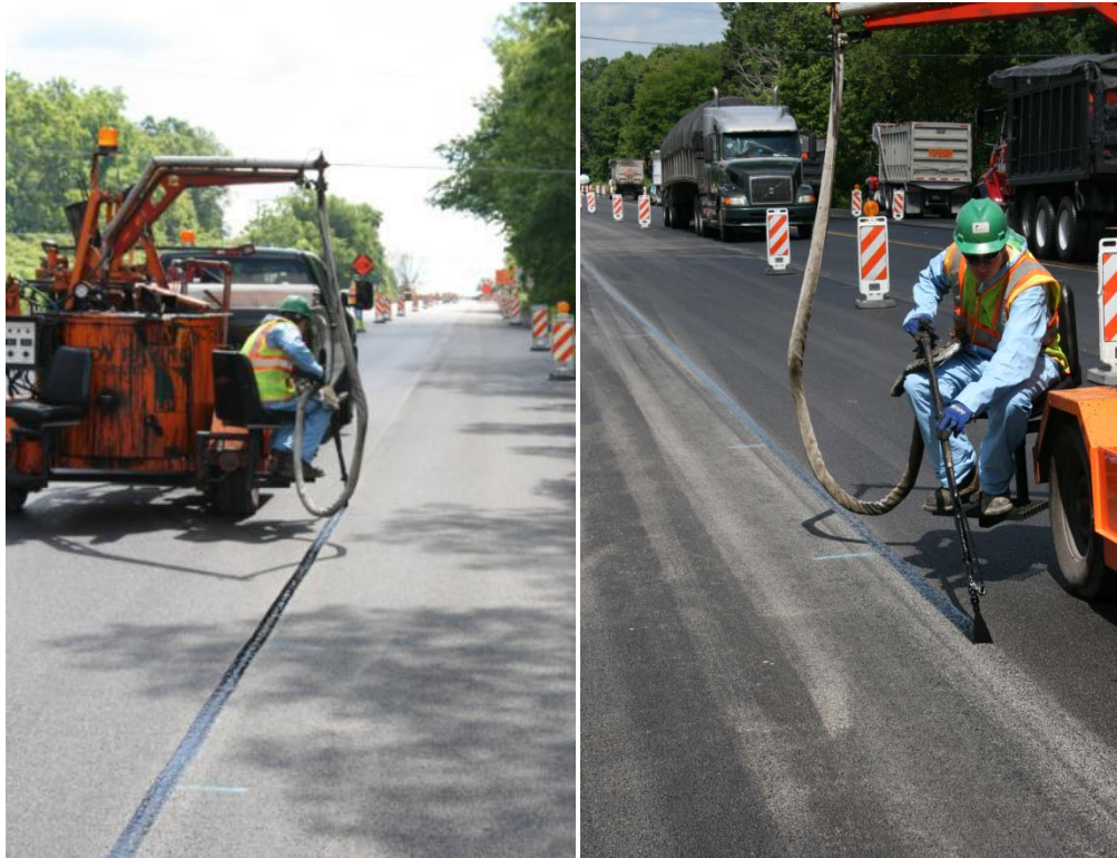
Figure 12. Overbanding Longitudinal Joints 4-inches Wide with PG Binder
