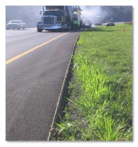
First Pass Must Be Straight! Unanimous that a string-line should be used to assure first pass is straight
