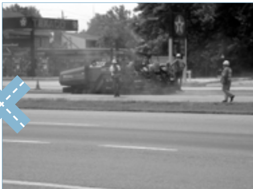
Replacing the PCC portion of the intersection with Superpave
