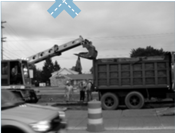
Removing the PCC portion of the intersection
