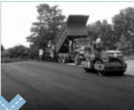
Preconstruction Trial Run
