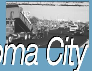
1987. The surface mix was a self-leveling mixture, placed with a prime coat, a tack coat, and a reinforcing fabric. "It served as a crack and rut filler," says Craig Moody, ODOT engineer. "We put it down at night and on the weekends and were able to get traffic on it in a matter of hours. "It went down fast and smooth," he adds. "The finished product, now 13 years old has performed well and has eliminated road chatter."
