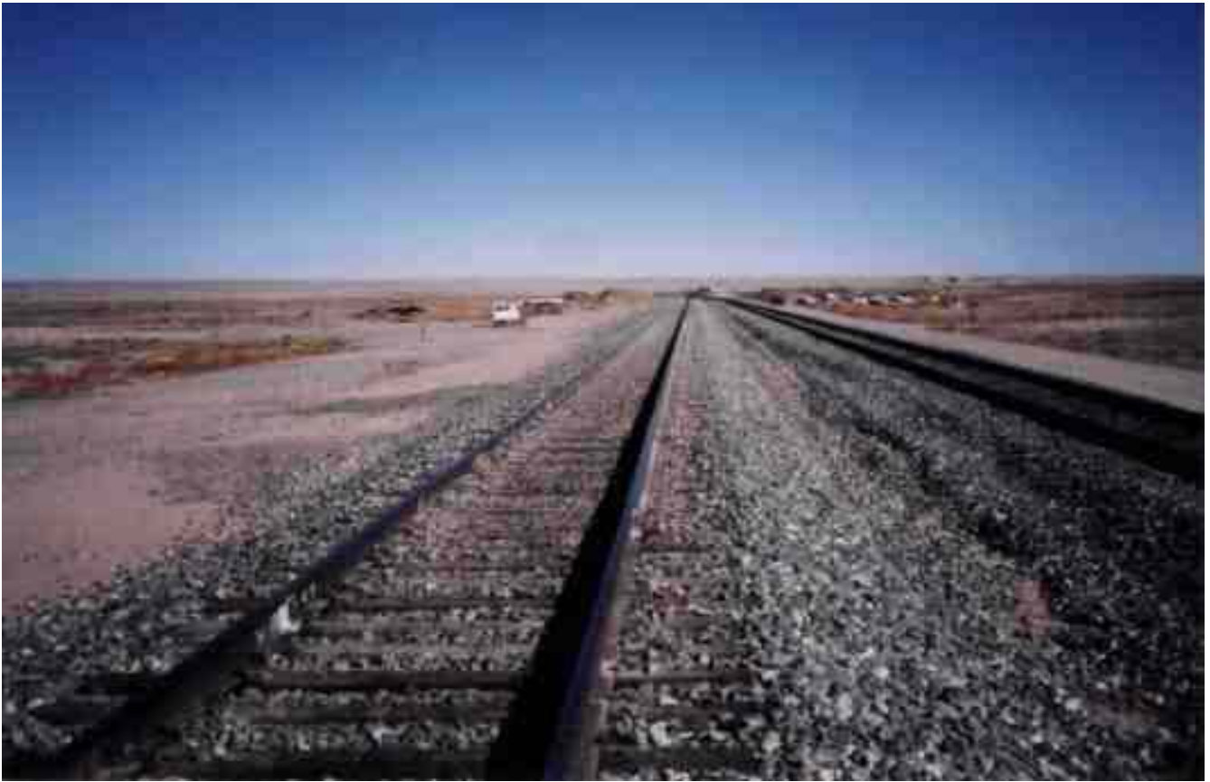
Completed Test Section Graphic Figure 1
